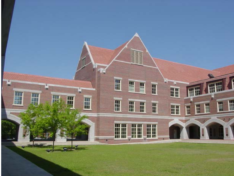
PHOTO 3.16 Courtyard of the New College of Medicine at the site of the former Florida State University School (FSUS).
